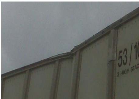
Complete failure of the same intermodal box in transit
